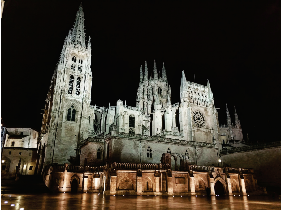
Figure 1.1. Burgos Cathedral, Spain. Night-time illumination, stained-glass windows.
